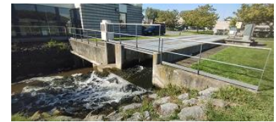
Effluent (after treatment)
