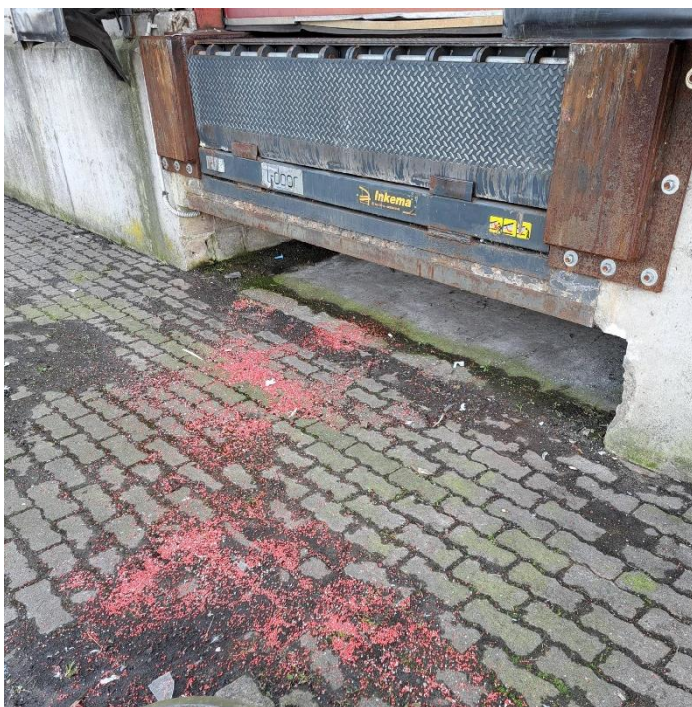
Pellets at the loading area
